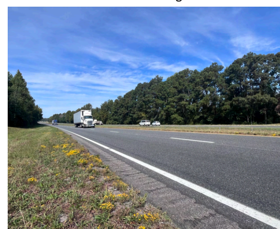
Pictured below: Microsurfacing on US 74
